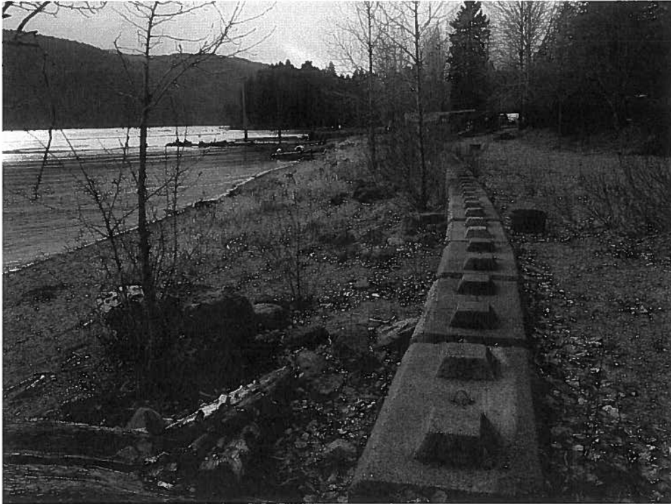
Photo 6. View west taken from the western edge of the campground study area showing day-use area that has been identified for riparian restoration plantings.
